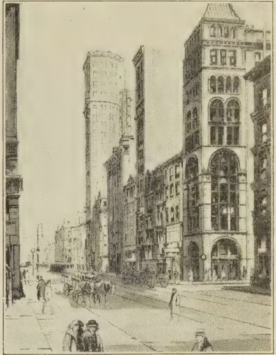
THE SAME SCENE AFTER THE OVERHEAD WIRES WERE REPLACED BY UNDERGROUND CABLES
